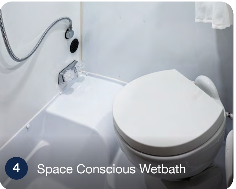
Lavvy, shower and toilet all efficiently utilized in one space.
